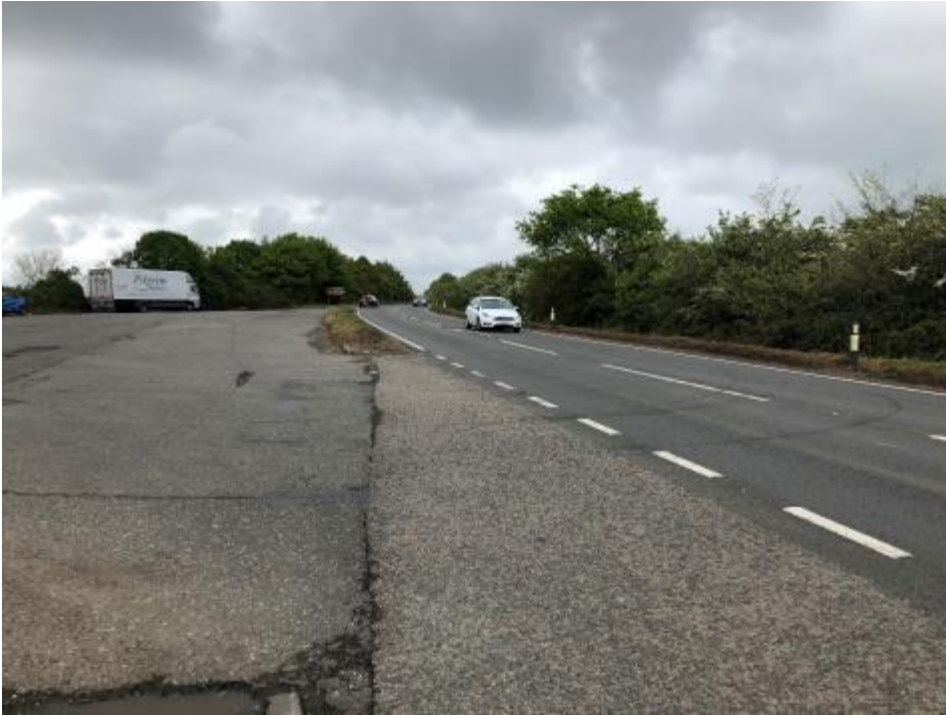
Photo 6 – A47 Main Road looking north
