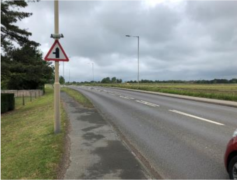
Photo 7 – A10 Main Road looking north
