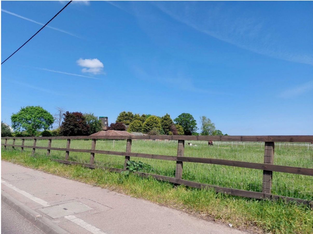
Plate 7 – The Mill at TF 6314 1678 as seen from A10, looking north-east
