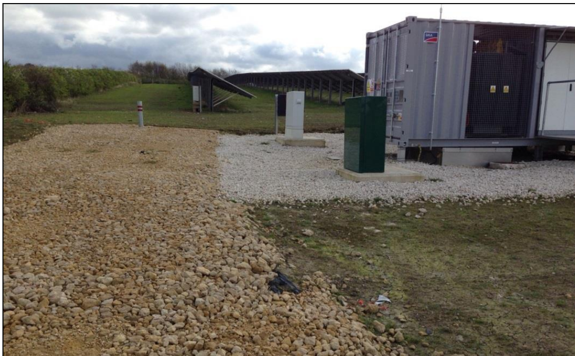
Plate 3: Typical Type 2 aggregate at a solar farm
