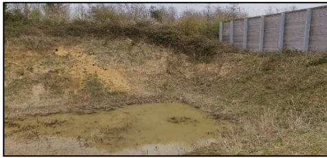
Photograph 1: Small attenuation basin (TN1)
