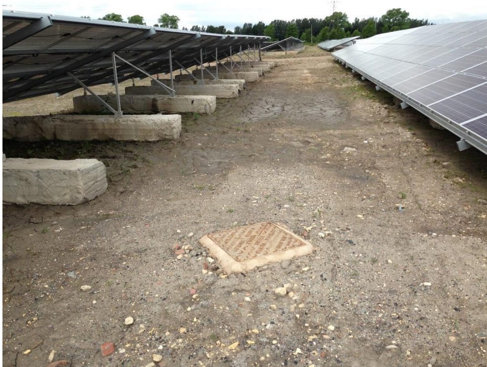
Plate 1: Typical concrete 'shoe' ballast system 57
