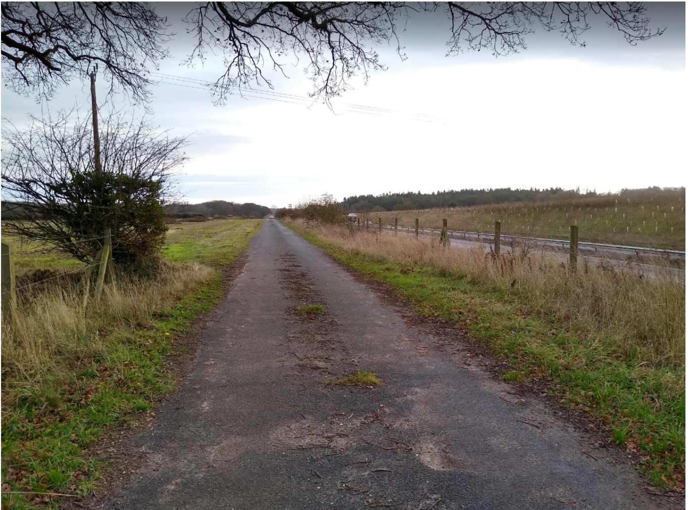
Figure 3 Existing access road looking east
