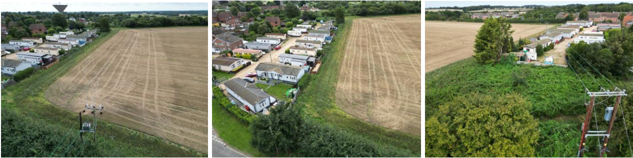
Figure 3-5 Overhead power lines at the north east side of the development site
