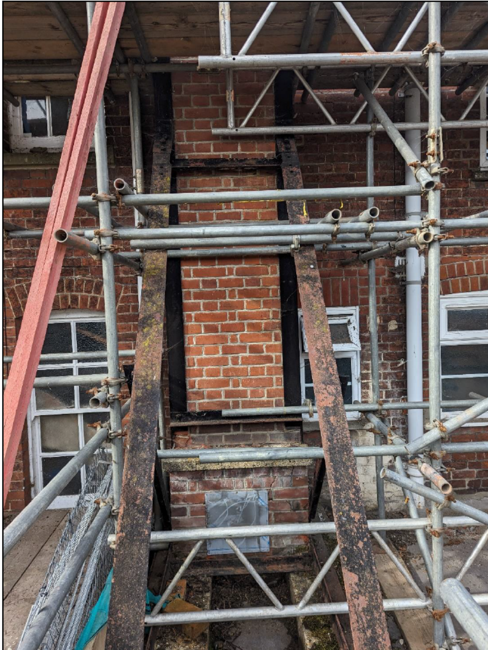
Image of the existing chimney and steel supports
