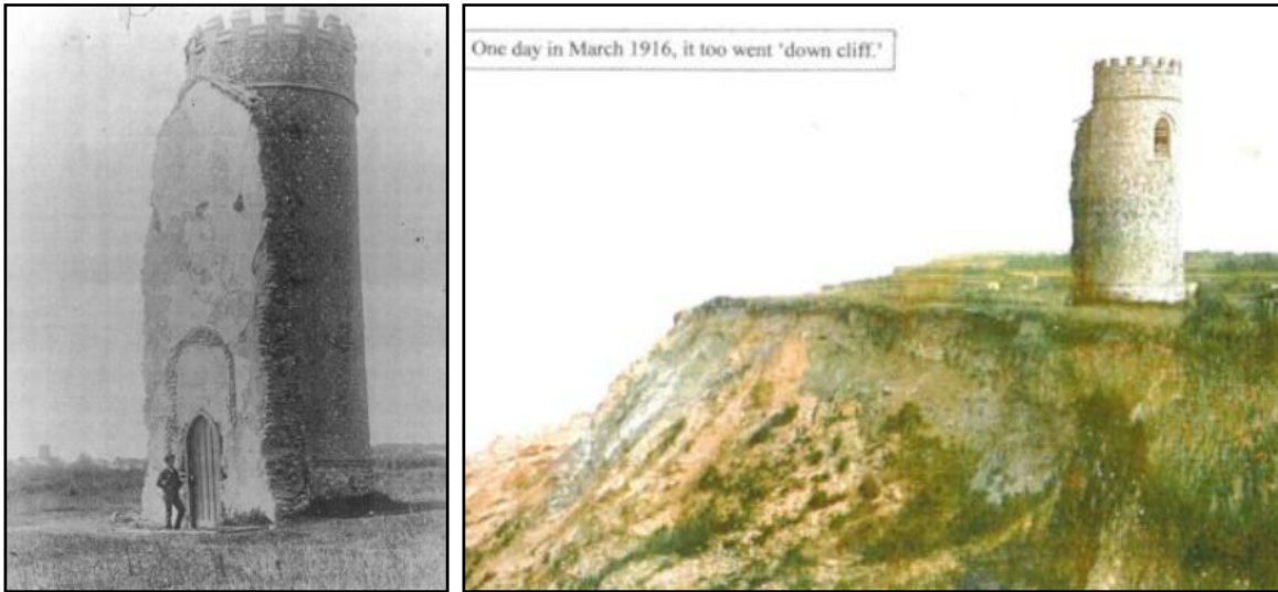
Historical depictions of the former church following storm damage
