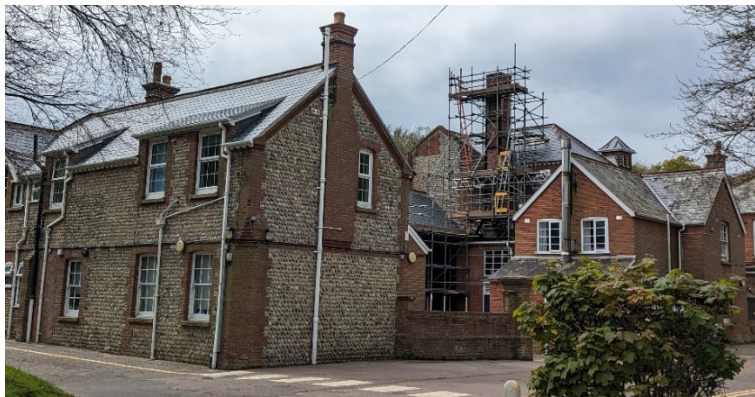
▲ View of chimney within courtyard
