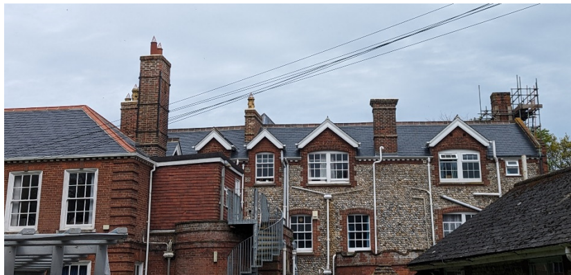
▲ Photo showing the adjacent chimney with steel bracing installed
