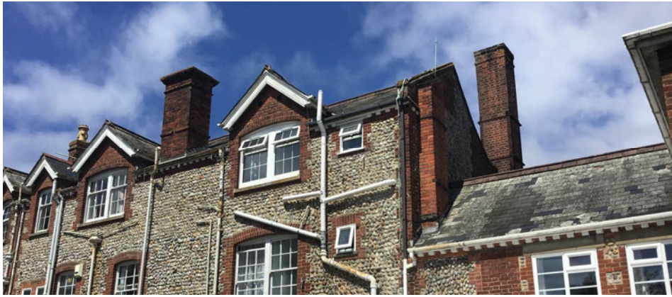
▲ Photo showing existing chimney and adjacent roofline
