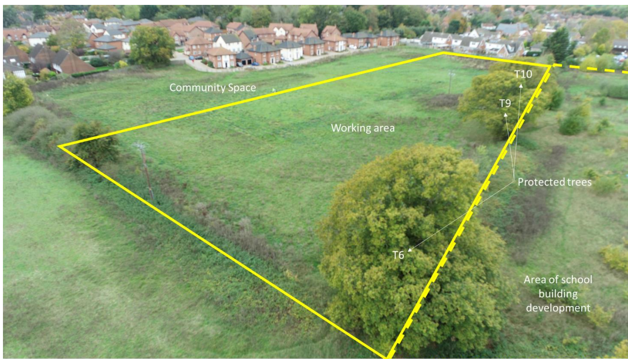
Figure 3-1 South westward view over the site
