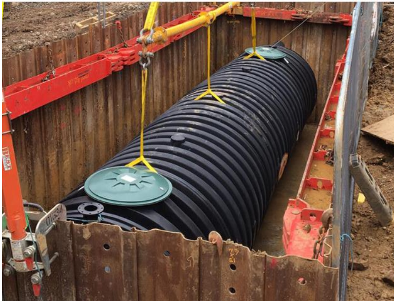
Graf Fire Water Tank Installation
