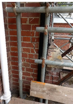
▲ Cracking to chimney structure
