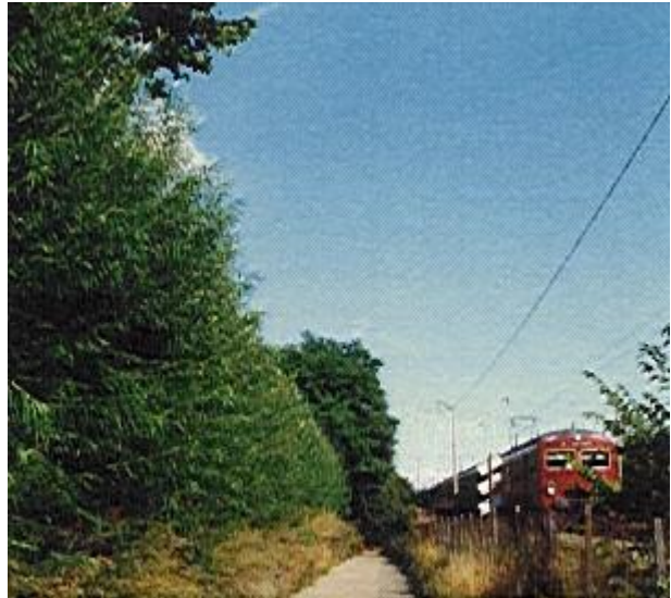
The living Green Barrier providing extremely effective noise abatement from train tracks next to a housing area.
