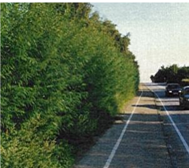
The Green Barrier in living willow erected as an acoustic barrier between a busy road and a primary school. Spring re-growth after winter trimming.
