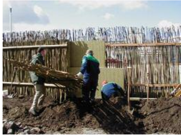
Single units are delivered, ready for construction. Sound barriers do however need to be erected by professionals.
