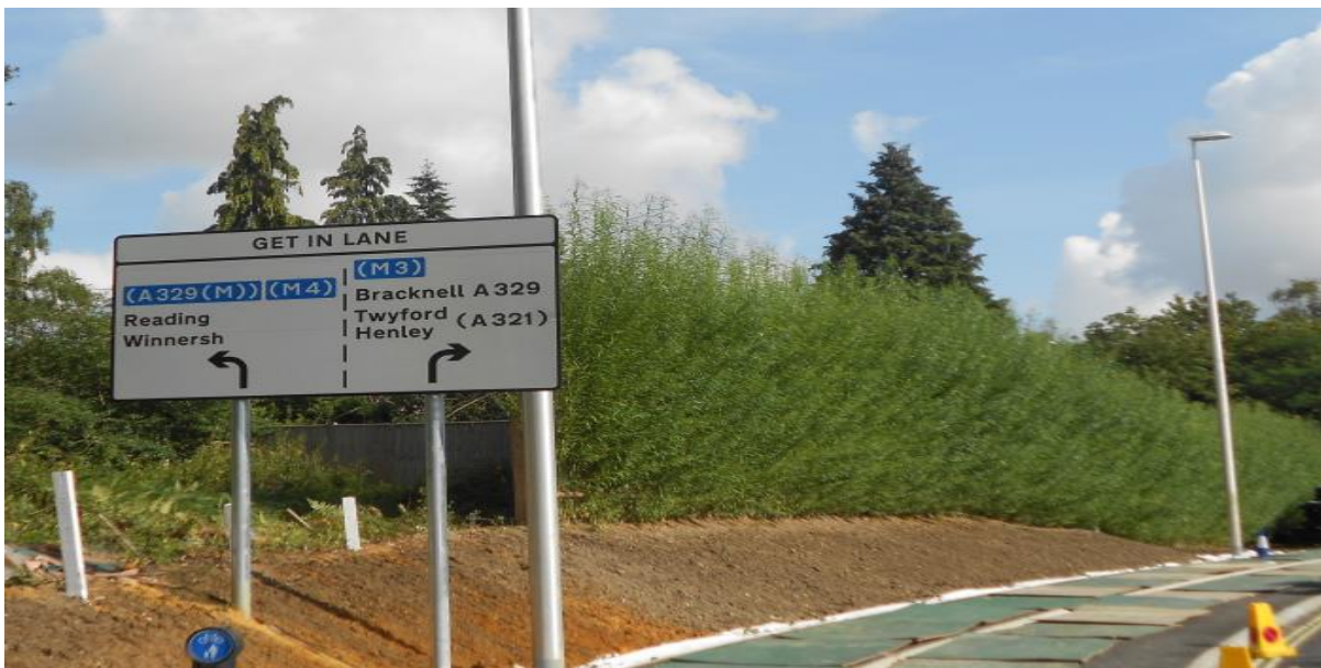
Living acoustic fencing 6 months after installation
