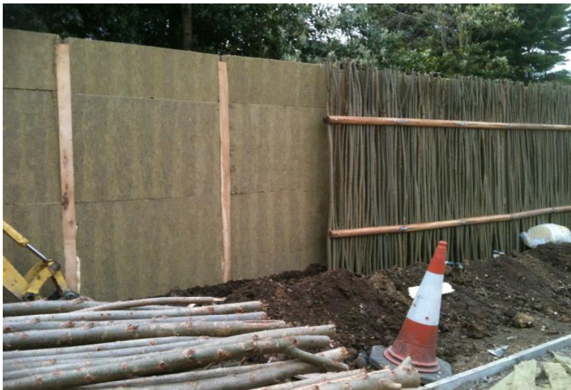
Components of the living acoustic fencing visible during construction
