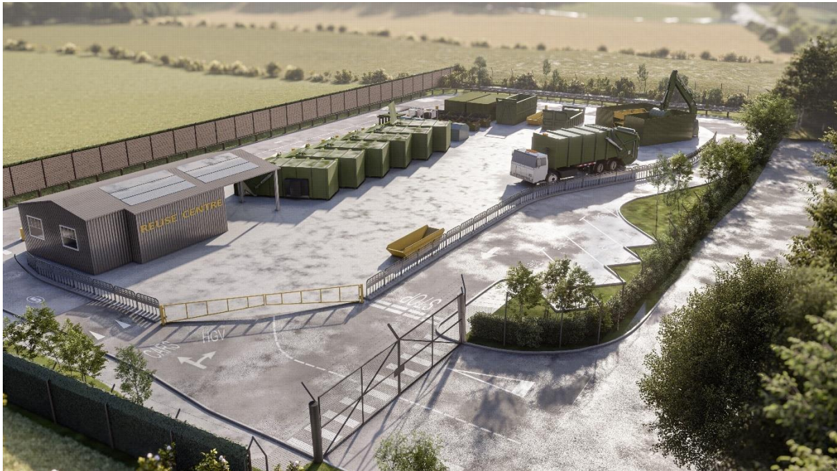
Figure 15 Showing Entrance / Exit gate. The gated central area is exclusively for authorised HGV movements for container servicing. Four Staff Only car parking bays and the site exit route shown mid right of image.
